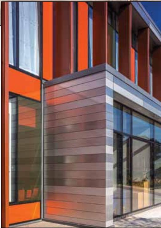
Aluminium is also highly reflective, making it very efficient for light management, and energy saving. Aluminium ventilated cladding protects the outer side of insulation materials against rain, which could cause their heat-saving properties to deteriorate. The air gap also helps to retain warmth, making it possible to prevent considerable loss of energy from a building.
